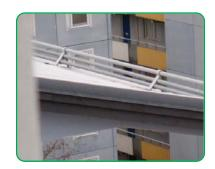
The source of PIM was in this case a corroded snow fence. Without DTP this source of PIM would have been almost impossible to locate.
